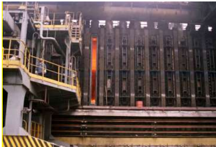
Fig.1. Coke oven battery (front-side view)
