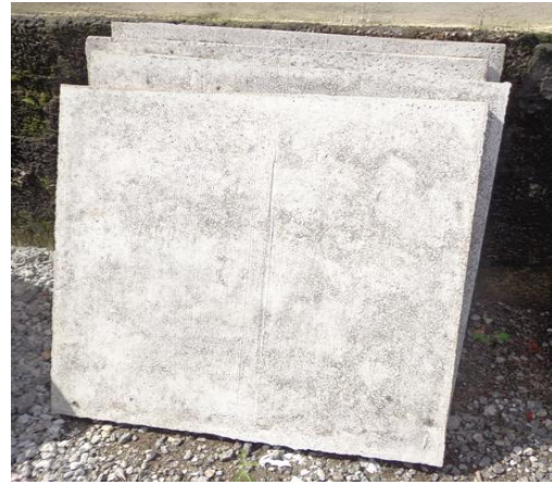
Fig.2: Finished slabs placed for curing
