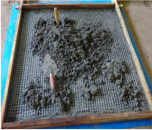
Fig.1: Casting of Slab
