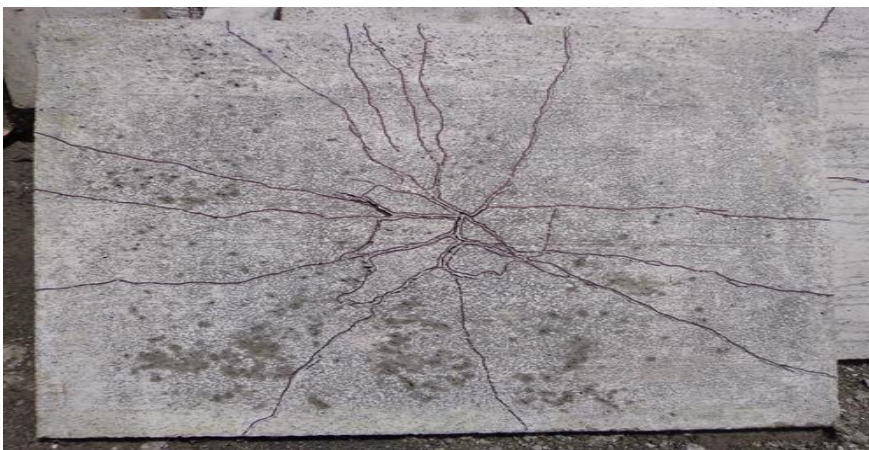
Fig.6: Crack pattern in slab with double layers of wire mesh
