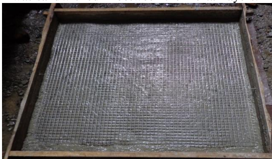
Fig.1: Casting of Wall panel
