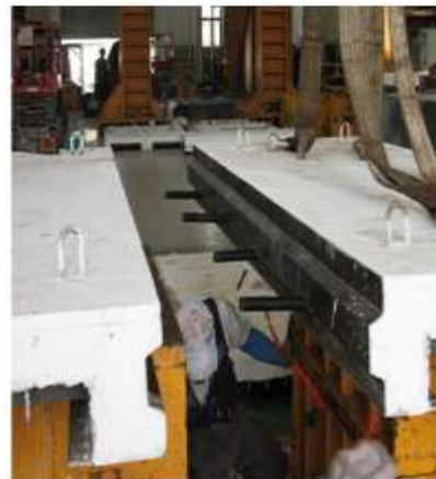
Fig. 5: Assemblage of deck [7]
