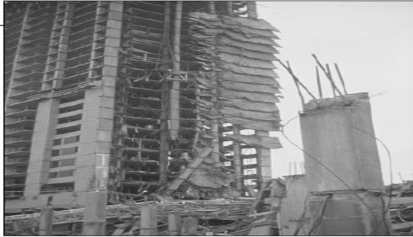
Figure 4: Collapse of Skyline Plaza
