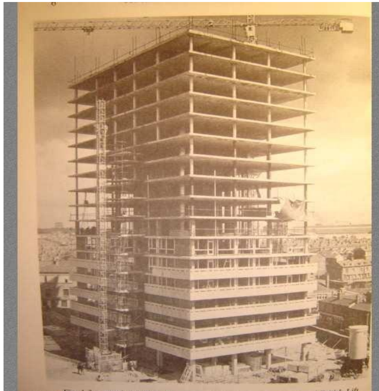
Figure 2: Reinforced concrete flat slab building
