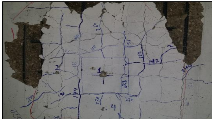
Figure (25): the crack pattern and mode of failure of specimen "SC".
