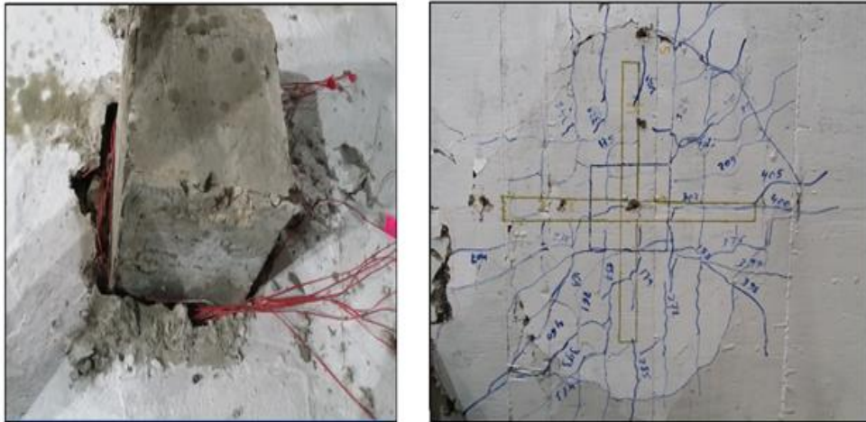
Figure (26): The crack pattern and mode of failure at the top and bottom of specimen "S-L1-2"
