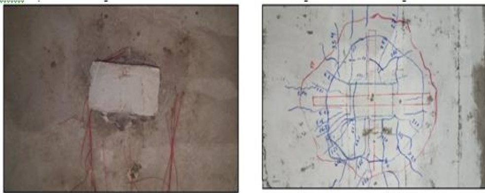
Figure (30): the crack pattern and mode of failure at the top and bottom of specimen "R-L1-2-45".
