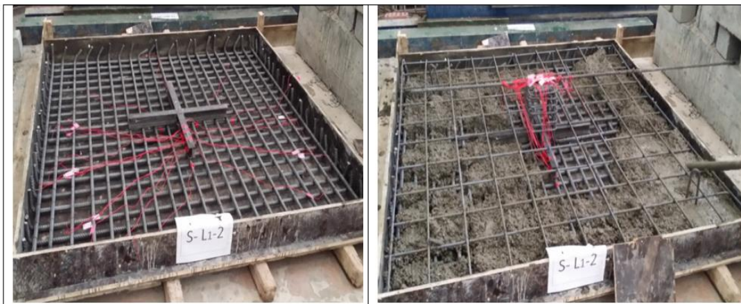
Figure (6): specimen "S-L1-2" during preparing and placing of concrete in lab.
