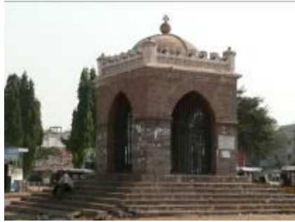
Fig. 11. Queen Victoria Pavilion
