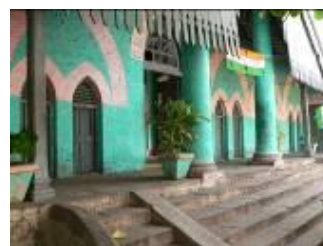
Fig. 10. View of the arches
