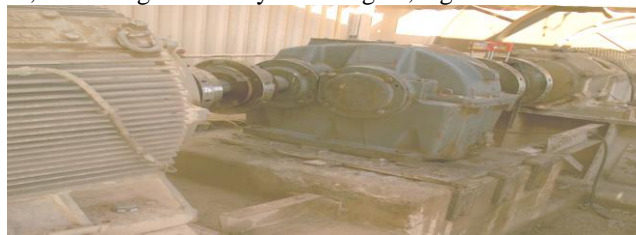
Figure 3: control fan equipment
