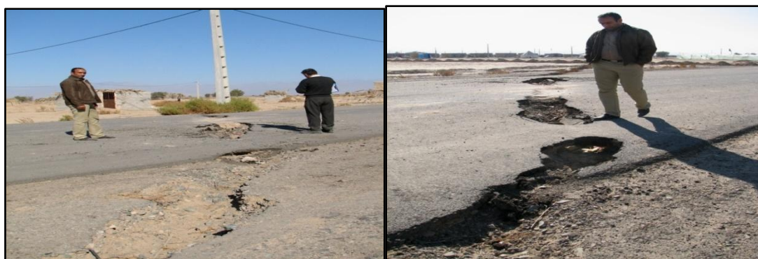
Fig. 10 Fissures in roads
