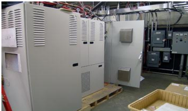
Fig. 1: High Voltage Power Supply (HVPS)
