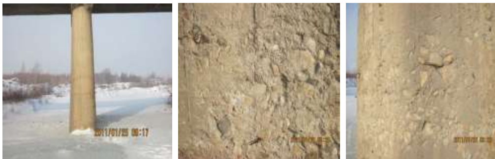
Fig. (11) Peel of the cement mortar and exposed gravels of pier condition
