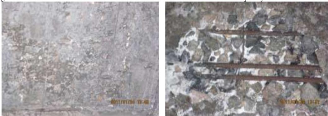
Fig. (20) The flange cracks, water seepage whitened condition and steel corrosion.
