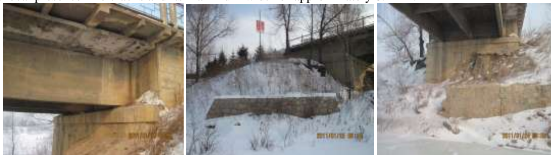
Fig. (10) Wing walls and ear wall damaged condition
