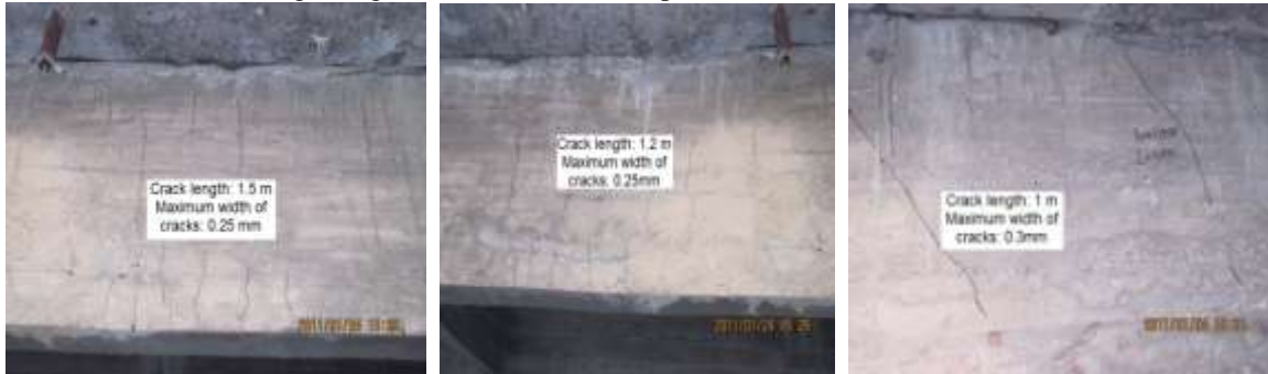
Fig. (17) Bending and diagonal tensile cracks pattern.
