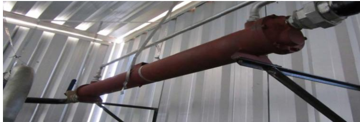
Fig. 4. Single-pass shell-and-tube heat exchanger Apema TST 175-5-1-A
