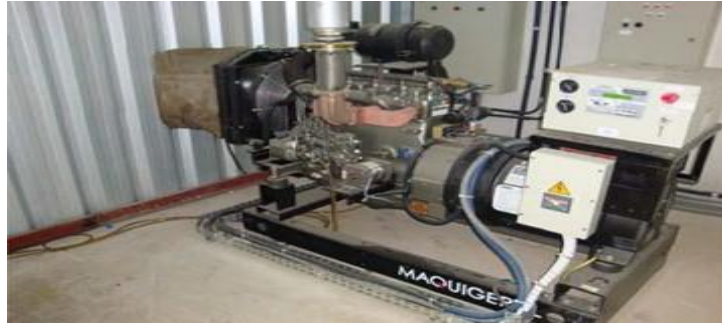
Fig. 3. GENSET installed in NPDEAS-UFPR
