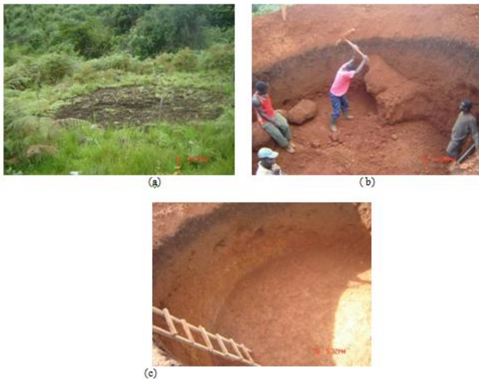
Figure 4: Some stages of excavation: (a) area to be excavated, (b) execution of works, (c) end of excavation
