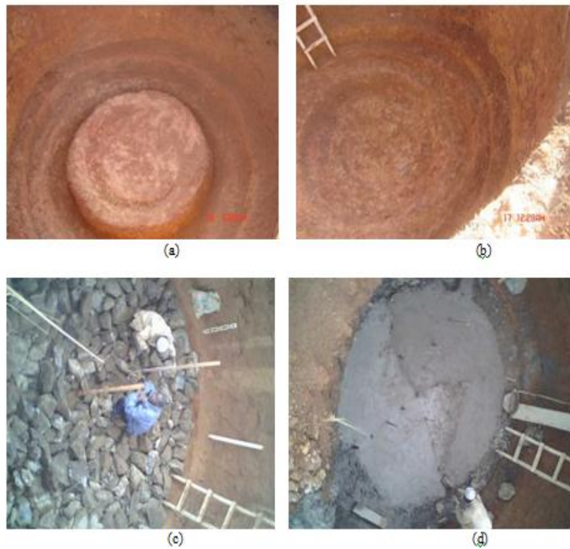
Figure 5: Different step of the foundation: (a) and (b)-transformation of the base, (c)- ruffle the strike in the conical shape, (d)- layout of the floor slab.
