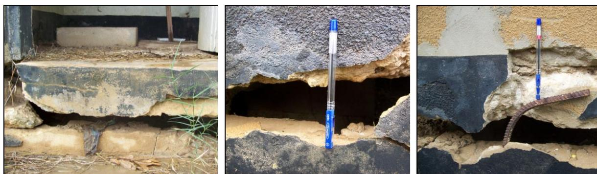
Figure 1: Cracks in buildings caused by expansive soil at Tumbi, Kibaha
