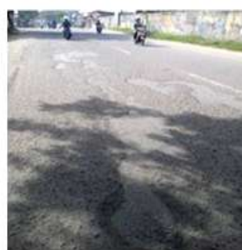
Figure 2.3. Sta: 0 + 500 (Exfoliation of the Surface Layer)
