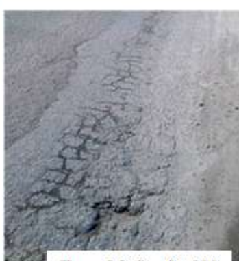
Figure 2.2. Sta: 0 + 300 (Alligator Cracking)
