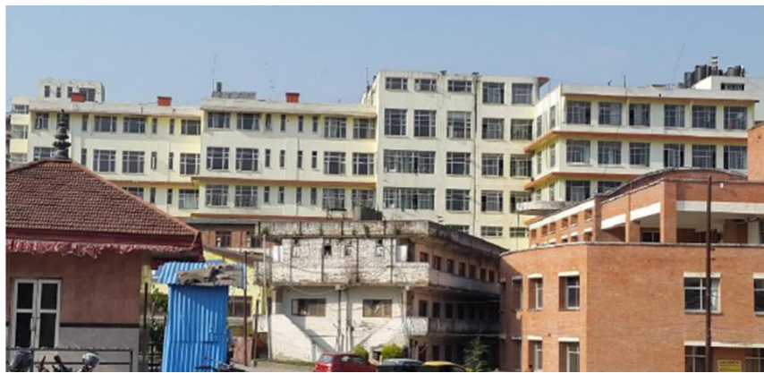
Fig.1. Front View of Existing Six Storey Hospital Building
