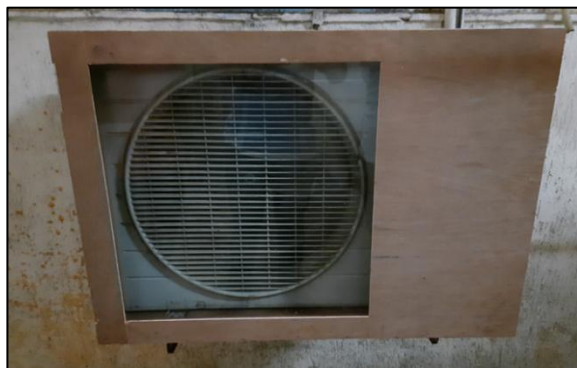
Figure 7: Outside box of the Waste Heat Recovery System
