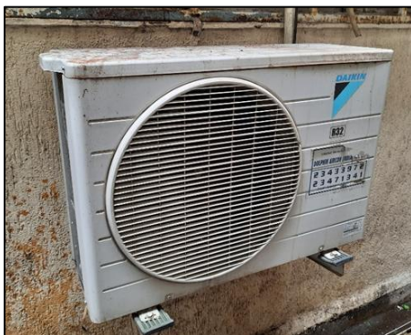
Figure 6: Condenser of Air Conditioner.
