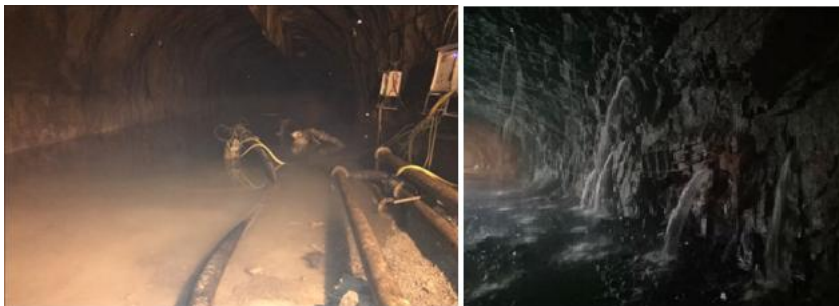
Figure 3: Tunnel flooding and water ingress
