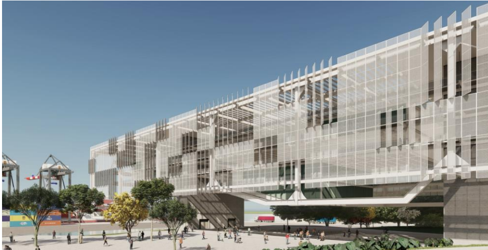
Figure 3 – Front facade of the building.
