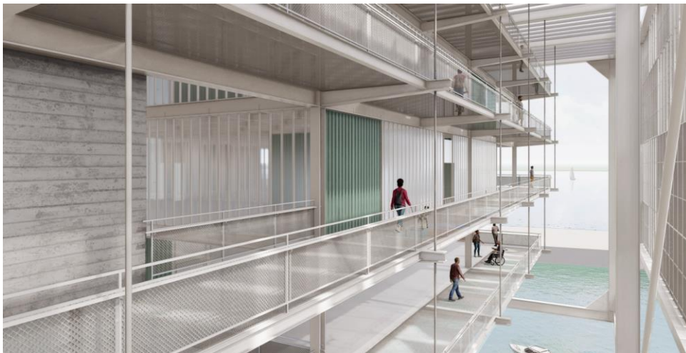
Figure 4 – Detail of the complex's metallic structure.
