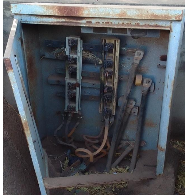
Figure 5. Broken dual pole in service. Figure 6. Under sized 415V Bus bar in service using wrong size of fuse in addition to birds nest behind the left unit at the top.
