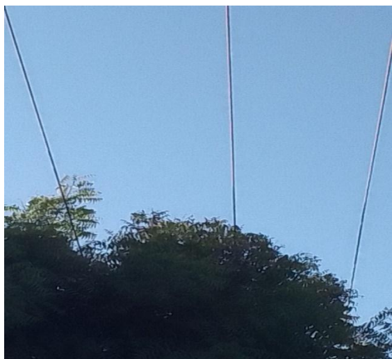
Figure 13. Tree in direct contact with high tension Line.
