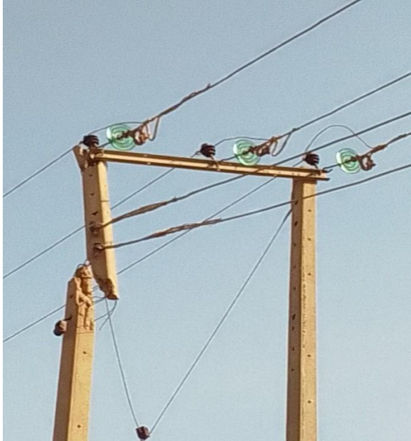
Figure 5. Broken dual pole in service. Figure 6. Under sized 415V Bus bar in service using wrong size of fuse in addition to birds nest behind the left unit at the top.
