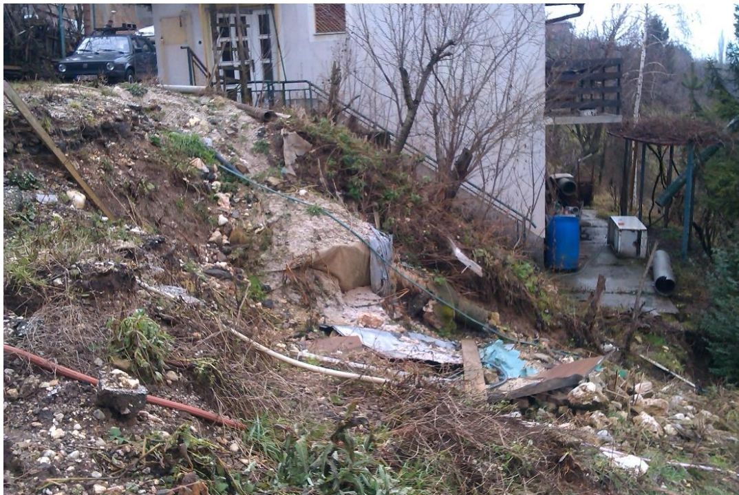
Figure 1. Part of the slope and developed area at the site (from the design documentation).
